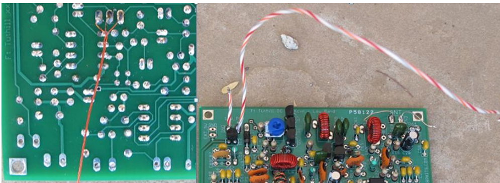
Figure 37. 3” R11 volume control wires on bottom, short ground and long 12v wires on top
